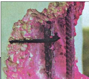
Typical carbonation test result
